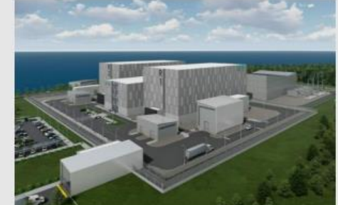
IMSR, Terrestrial Energy's avansert SMR
